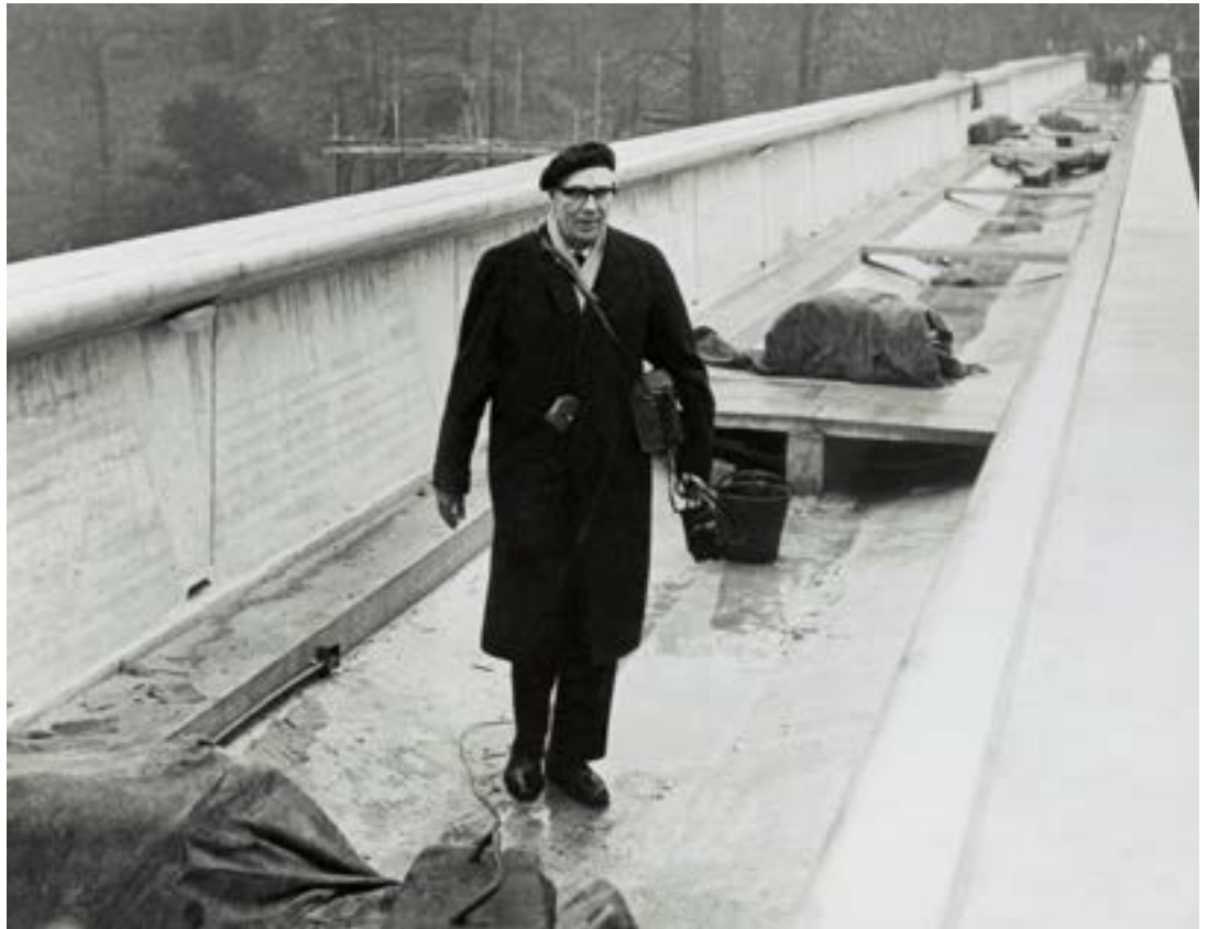
Sir Ove Arup pictured on Kingsgate Footbridge, Durham, 1963
